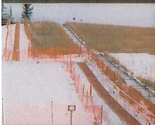
Tuff Step provides safe temporary working access to most sloped surfaces where anchoring is possible. May be used as individual stairs or joined together for longer runs. Possible uses include road/rail embankments, river banks, gravel pits, earth retaining walls, trenching, access to accident sites, construction sites, vehicles, general hilly terrain and temporary access between building levels. Can also provide safe temporary bridging over small holes and uneven terrain.
