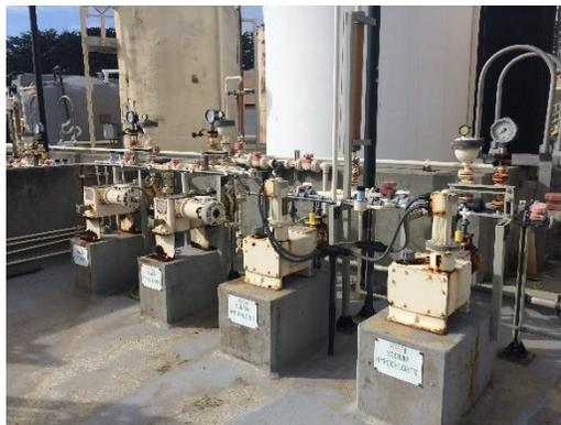
This project calls for the systematic replacement of the pumps, piping, heat tracing, and other badly deteriorated components in the chemical pump containment area. Existing power distribution and controls will be re-used with the new replacement equipment. To protect the new equipment from the sun and rain, a pre-engineered fabric sun shield will be erected above the containment area walls. The sun shield will also protect SAM staff while they maintain the pumps and equipment in this area.
